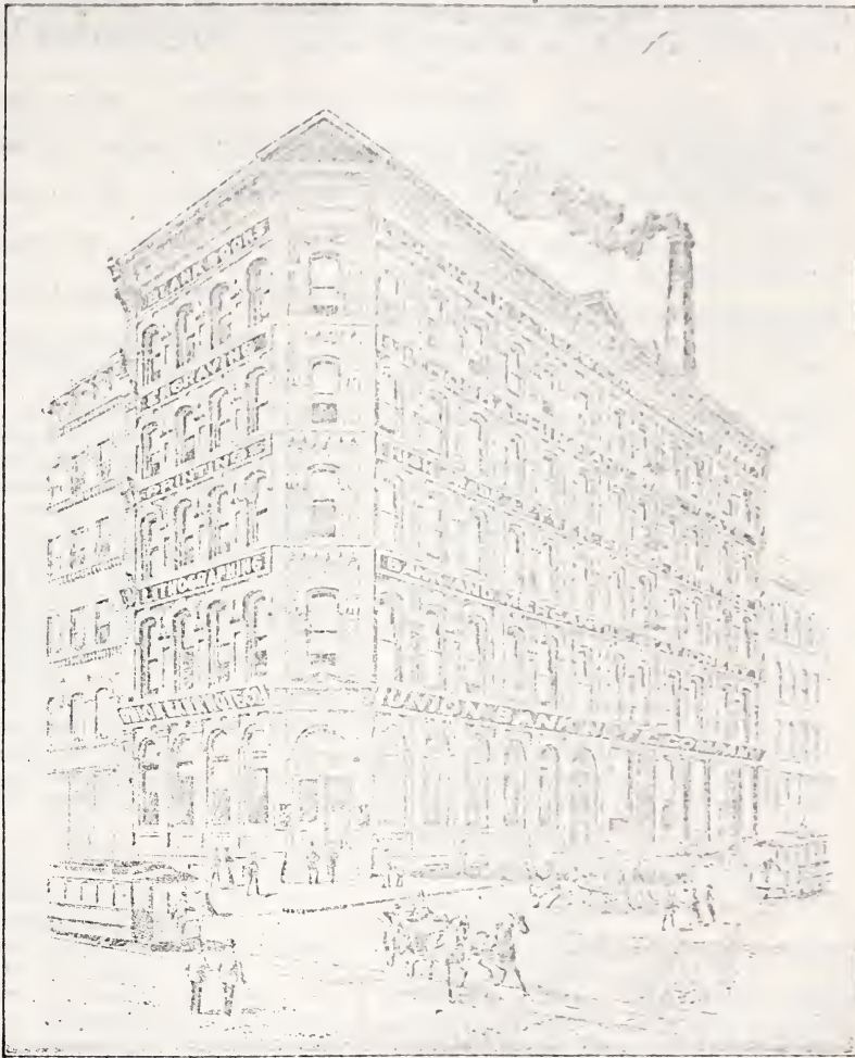
Our Factory, 600 Delaware Street, Kansas City, Mo.
